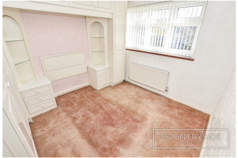
Upvc windows to front aspect, carpet, artex ceiling, fitted wardrobes, radiator and power points.
